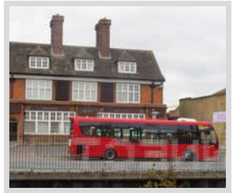
Head Office: Go-Ahead London Head Office: located on Merton High Street.
